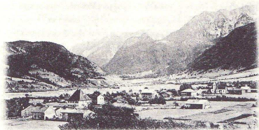
Gruss aus Pfronten-Ried.
